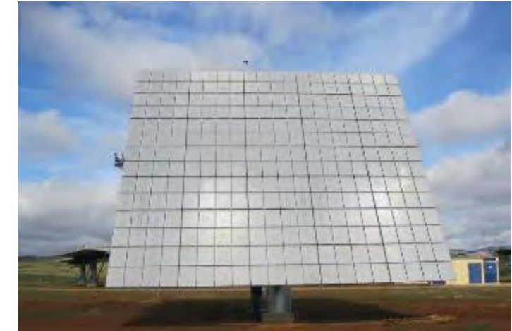
24.5 kW CPV system
