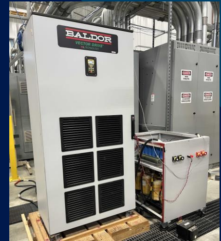
Baldor Vector Drive This 750 kVA Variable-Voltage Variable-Frequency Drive (VVVF) is used for medium voltage operation.
